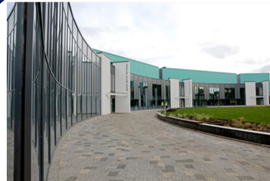
Temporary modular school building
